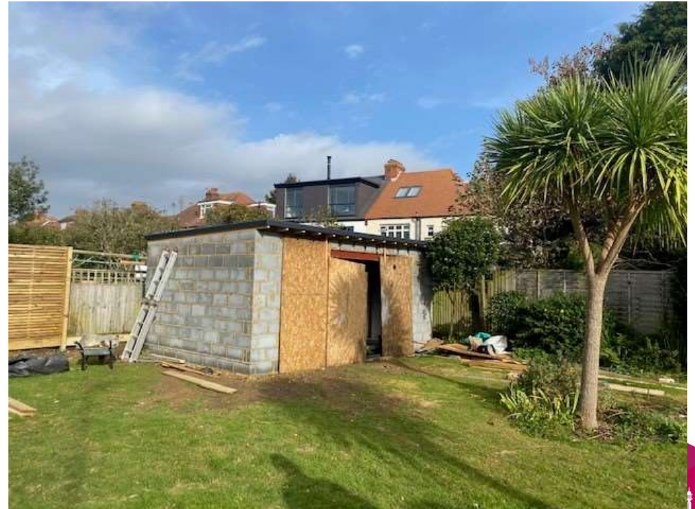
Outbuilding under construction under permitted development rights
