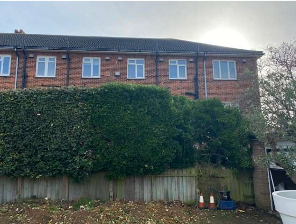
Southern boundary with Beverly Court flats
